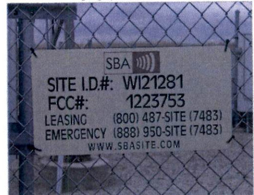
Exhibit 8-7 An example of appropriate tower signage placed on the security fence
