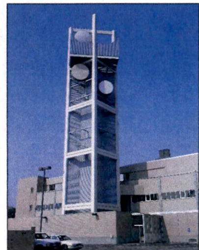
Microwave Tower in Oshkosh
